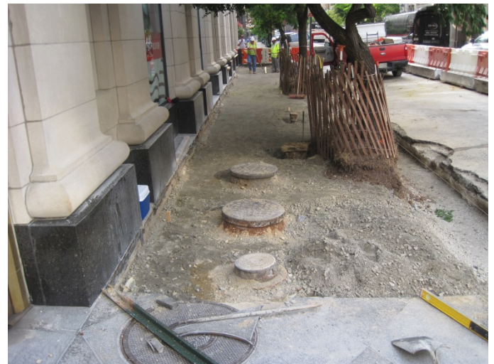
Sidewalk excavation at 1133 Connecticut Avenue going north
