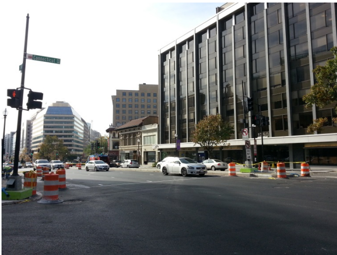
Completed paving on northbound Connecticut Avenue and N Street
