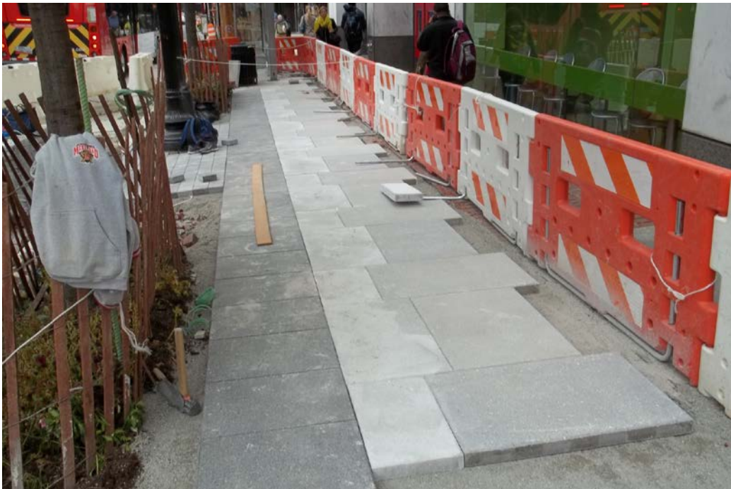
Reconstruction of the Sidewalk on the 1300 block of northbound Connecticut Avenue
