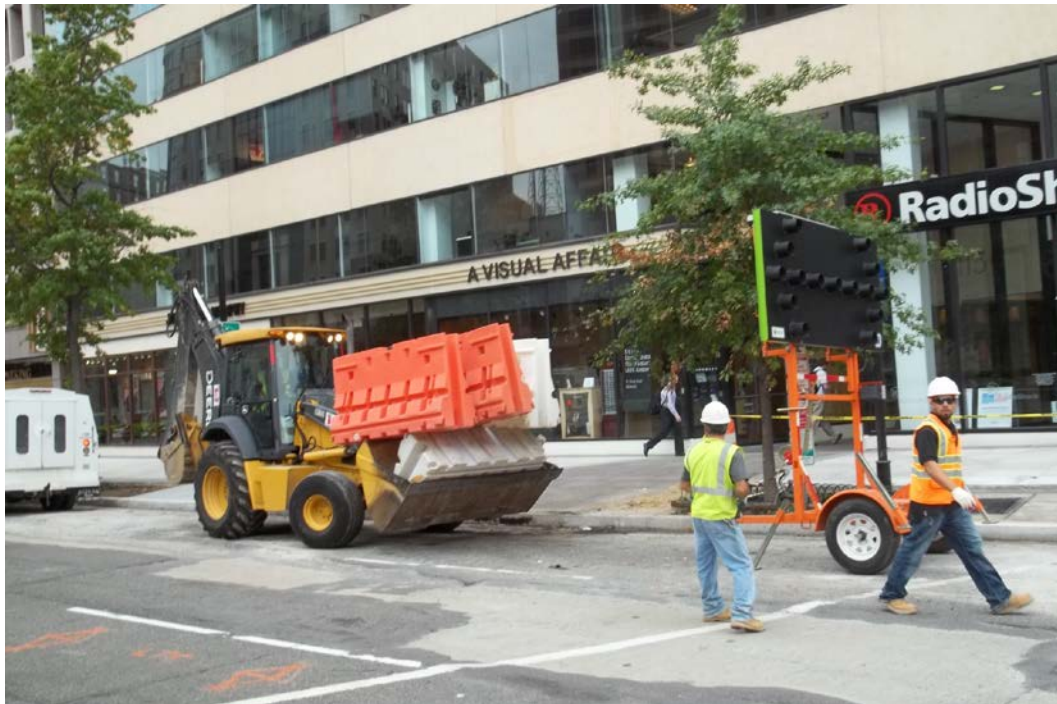
Cleaning the project and removing the water filled barriers.
