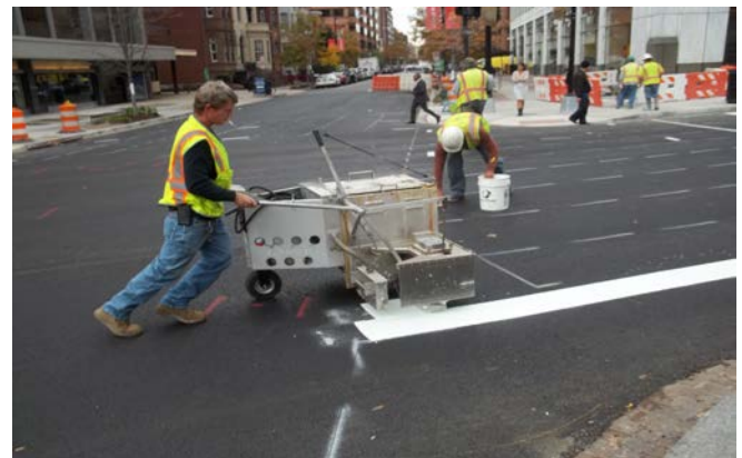
Road marking on the intersection of Connecticut Ave and N Street.
