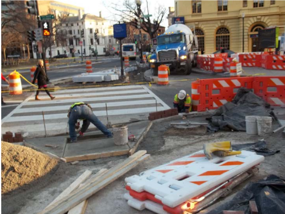
New handicapped ramp, located at the northeast corner, of the intersection between DuPont Circle and the southbound lanes of Connecticut Avenue.
