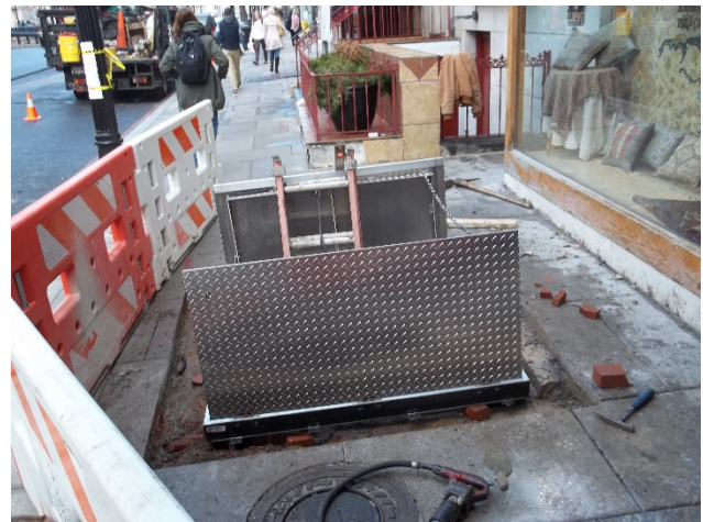
Installation of a vault gate along the 1300 Block of Connecticut Avenue
