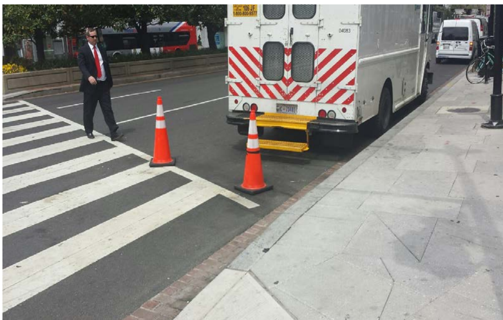
Safety cones are used to delineate a barrier between the service truck and the pedestrian crosswalk.
