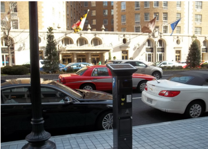
One of several new multi-space pay and display meters located throughout the Connecticut Avenue construction site.
