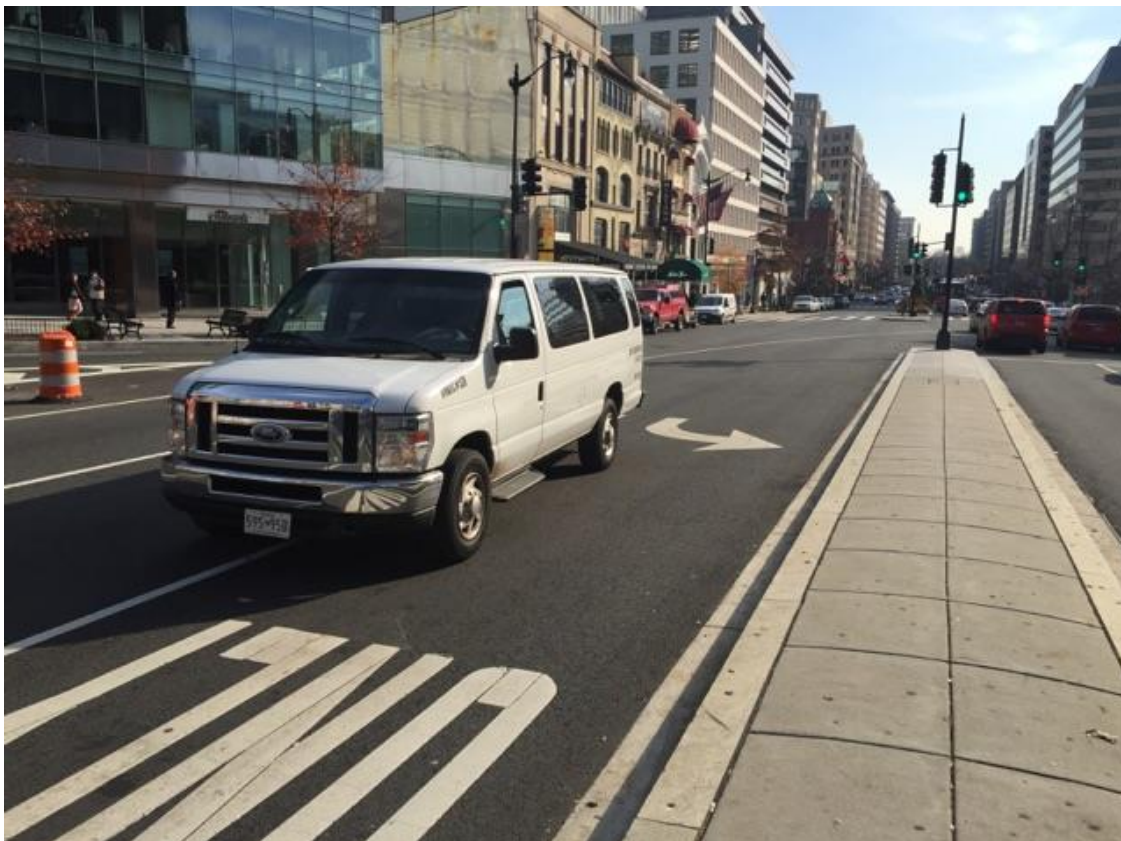
Volkert and contractor FMCC organize marking street light pole identification numbers.
