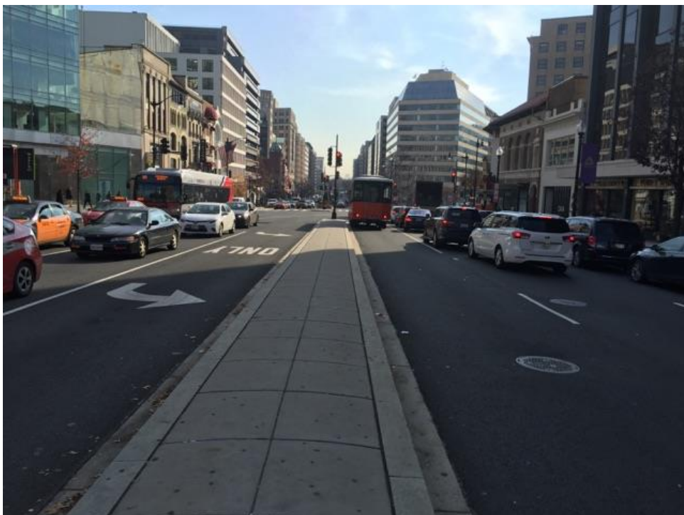
Maintenance of concrete paver sidewalks continues throughout the project.
