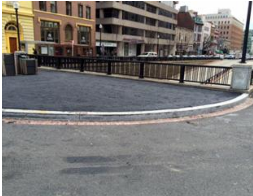
The completed temporary asphalt.
