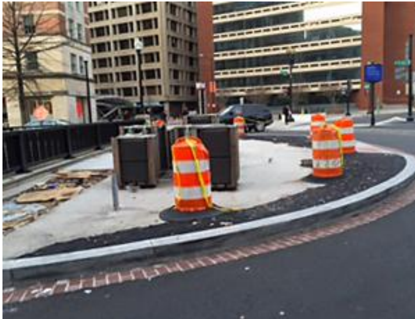
The condition of the overlook prior to asphalt placement.
