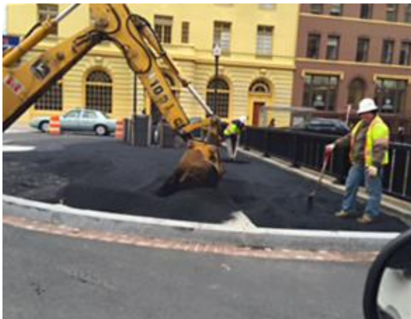
Placing the temporary asphalt at Dupont Circle located at the overlook.
